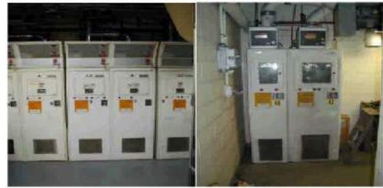
Figure 2. Silane gas cabinet
